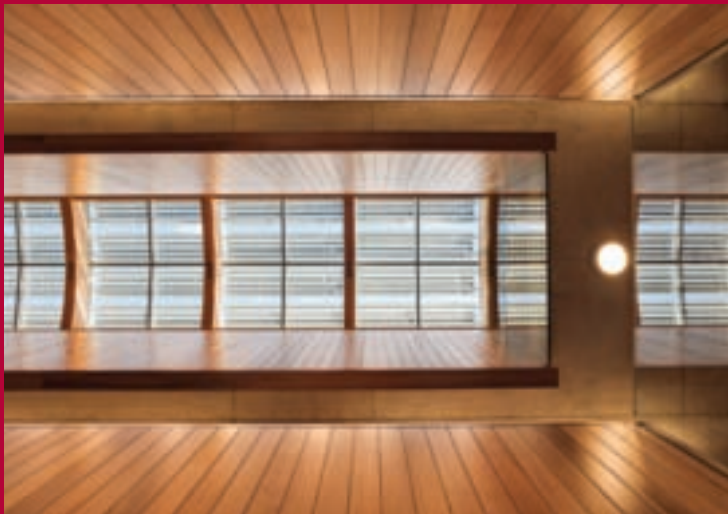
F. Looking up at photovoltaic panels embedded in glass in the building's skylight.
